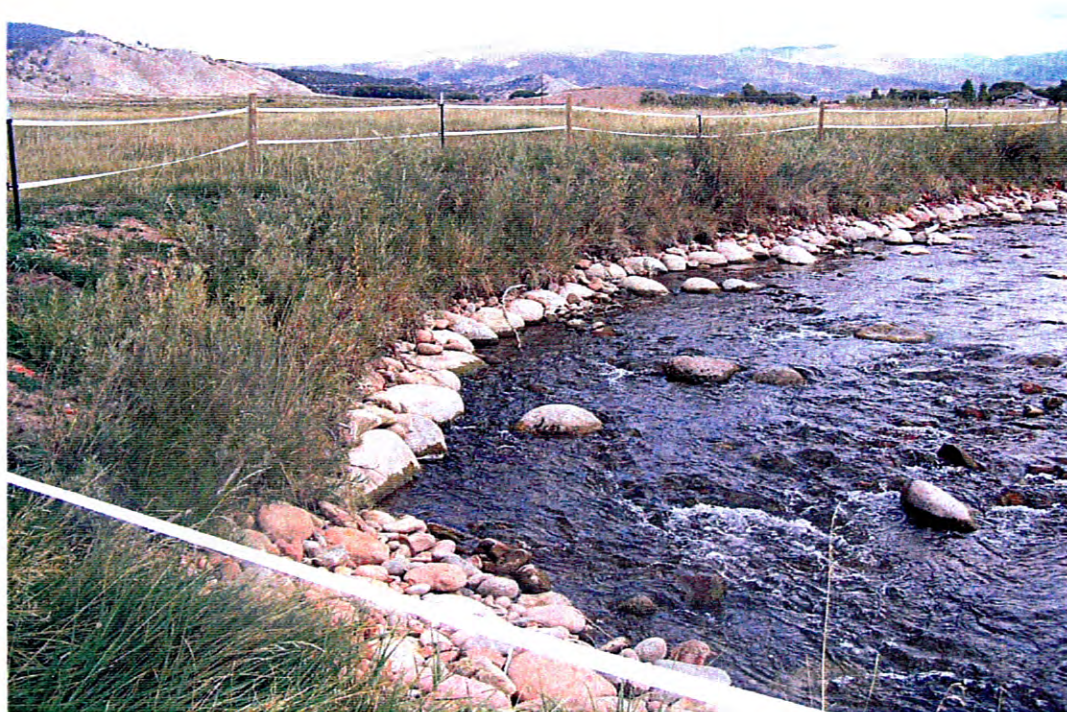
After Improvement Work: Bank Stabilized with Willows and Rock
