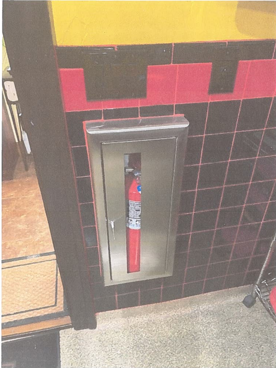
GARAGE MAIN LEVEL
