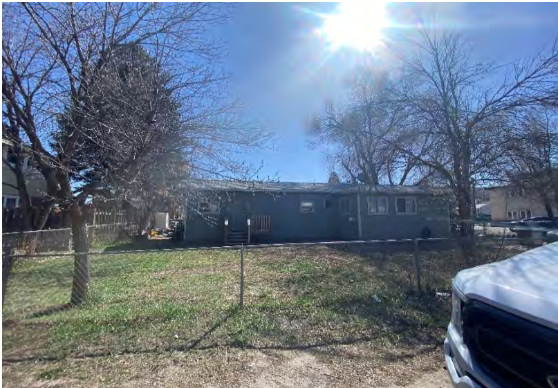
View of the residence at 130 Capitol Street. View to the west.
