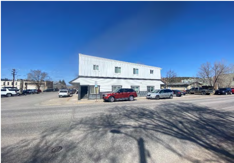
View of westerly adjoining Capitol Street, followed by multi-family residential. View to the west.
