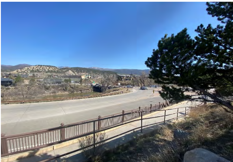
View of the northerly and northeasterly adjoining Grand Avenue, followed by the Eagle River. View to the northeast.
